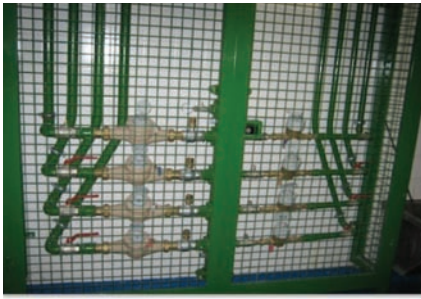
Water sectioning system used in a shopping center
