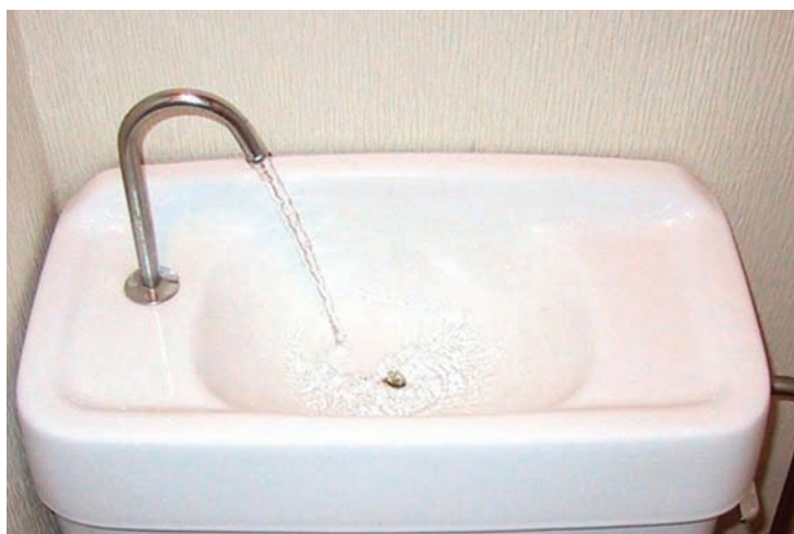
Water saving device on the Japanese toilet: Filling toilet flush tank while washing your hands
