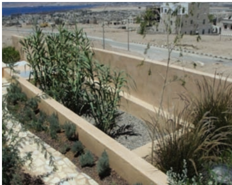
The wetland (filter bed) after 6 months of operation. The grass and bamboo started to grow
