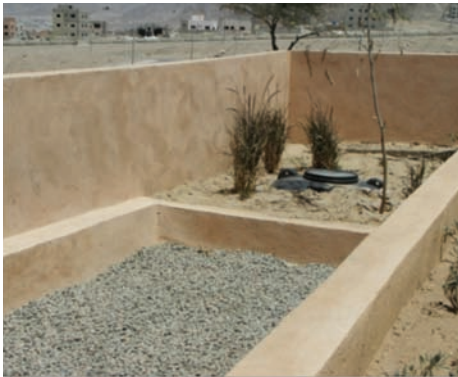
The settling barrel (back) and the horizontal flow constructed wetland (sand filter) (front)
