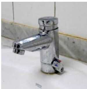
A push-button automatic shut-off tap system
