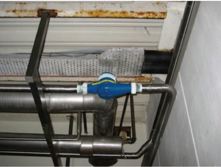
New water meter installed
